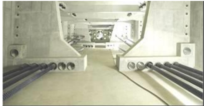
External ductless cables inside girder
