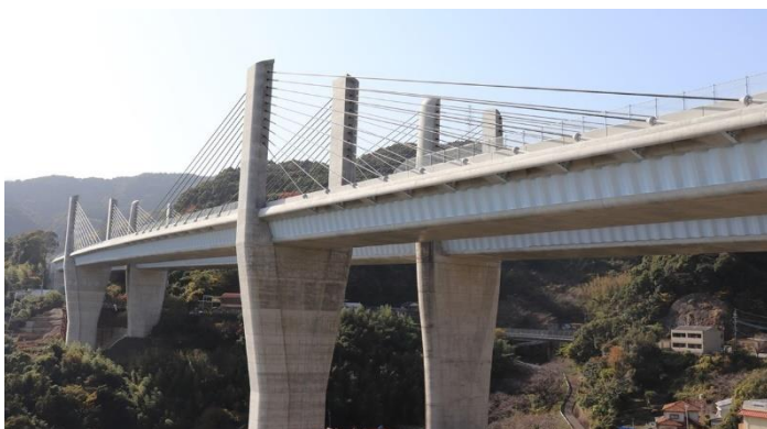
Himiyume Bridge (2019, Japan)
