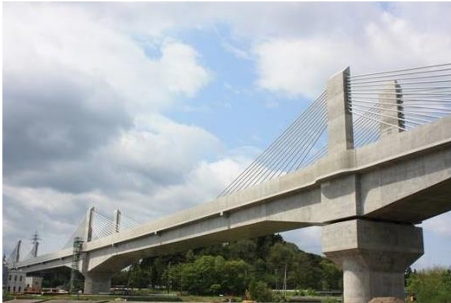
ECS stay cables at Sannaimaruyama Bridge (Shinkansen High Speed Rail, Aomori, Japan)
