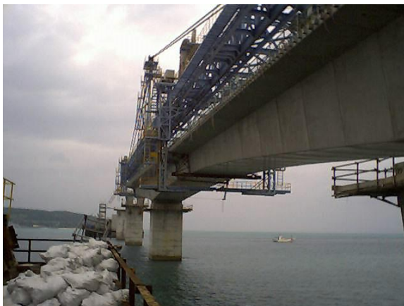
Kouri Bridge (Okinawa, Japan)
