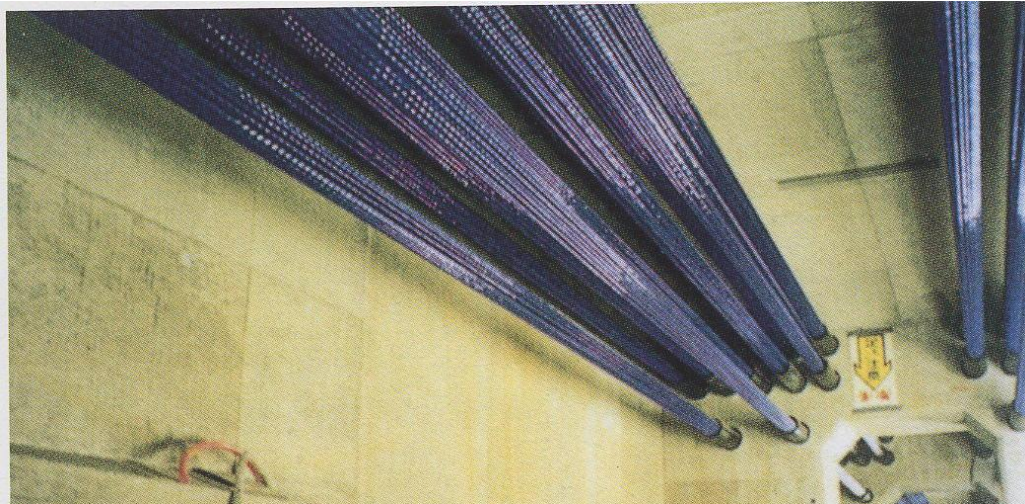
External ductless ECS cables inside of girder (Ikeda-hesokko Bridge: FLOGARD™)
