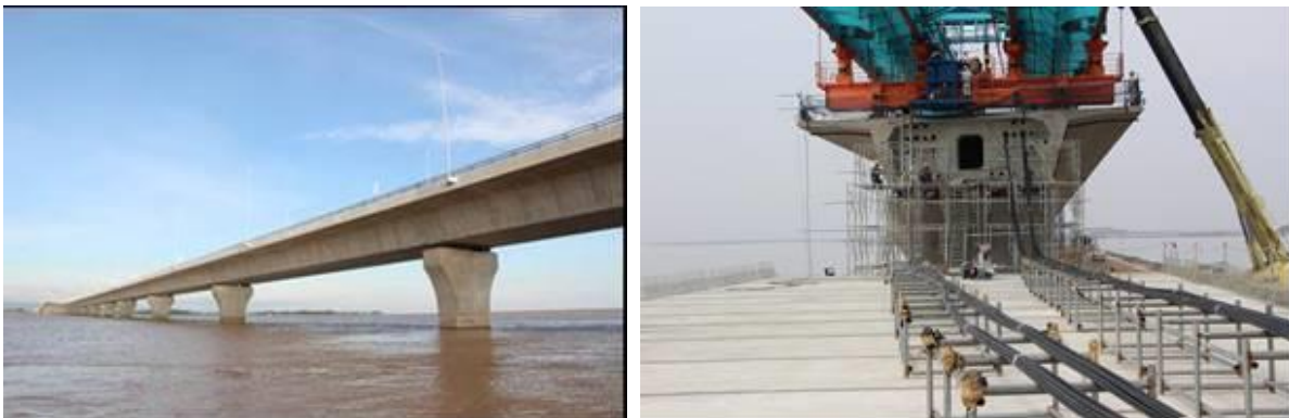
Example case of HDPE coated FLOGARD™ application for external ductless cables
