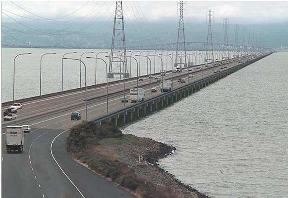
San Mateo Bridge (California, USA)
