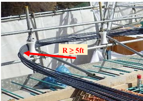
Deviation radius at installation (R≥5ft)
