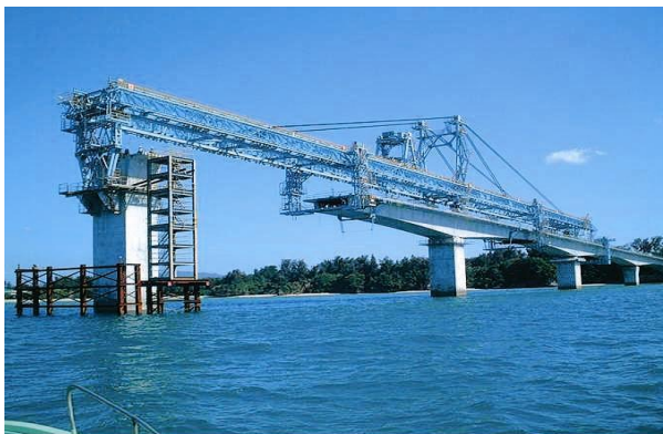
Internal cables in corrosive environment
